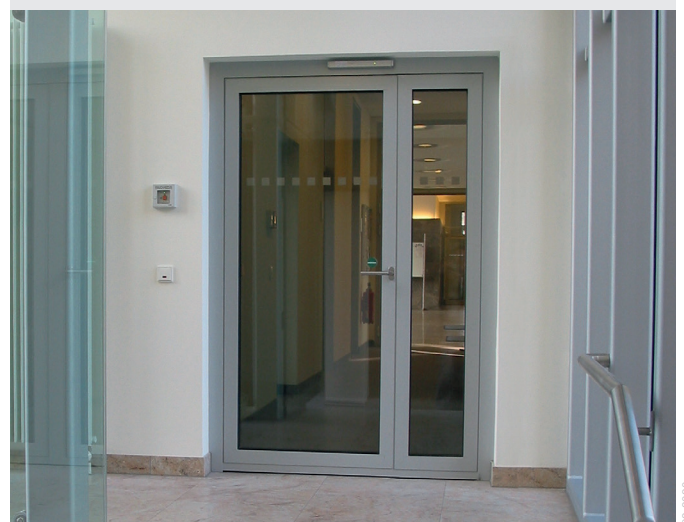
Hinged door, outward opening. Special frame with surrounding leaf profile and lowering gasket.
